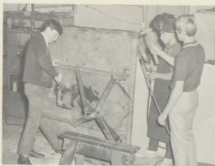
Randy Bridges, Mark Umberger and David Turner learn techniques of welding
